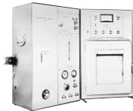
The **Model 154-D**. In this unit, the amplifier of the flame-ionization detector was incorporated in the upper part of the recorder cabinet (right). The rotary-type gas sampling valve, originally introduced with the Model 154-B, is mounted on the left side of the instrument cabinet.
